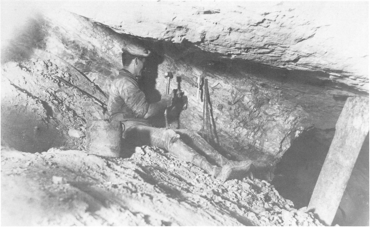
Single jacking was the earlier method of drilling in preparation for blasting. Photo courtesy California Bureau of Mines.
