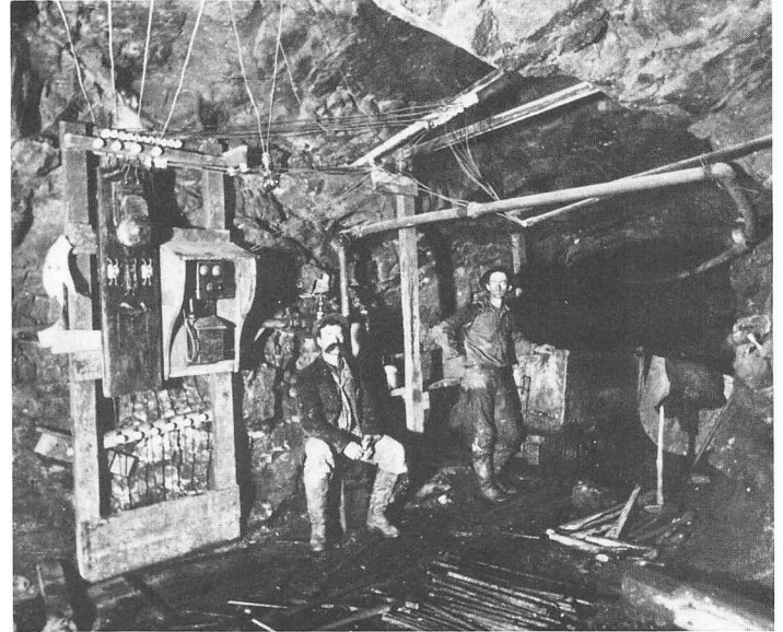
A hoisting station in a mine was the place where men, supplies, waste rock and ore were raised and lowered to various levels of the mine. The bell signal system, left, was a way to communicate with people in the mines. A certain number of “rings” had a specific meaning for miners. Photo courtesy California Bureau of Mines.
